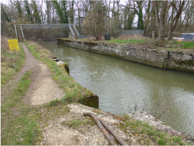
1. 1911–15 concrete lock chamber
