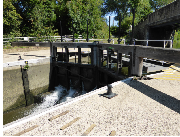
3. Head gates with modern gate paddles
