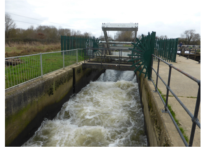
5. Sluice with radial gate
