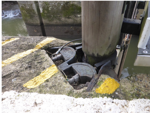
4. Head gate collar detail
