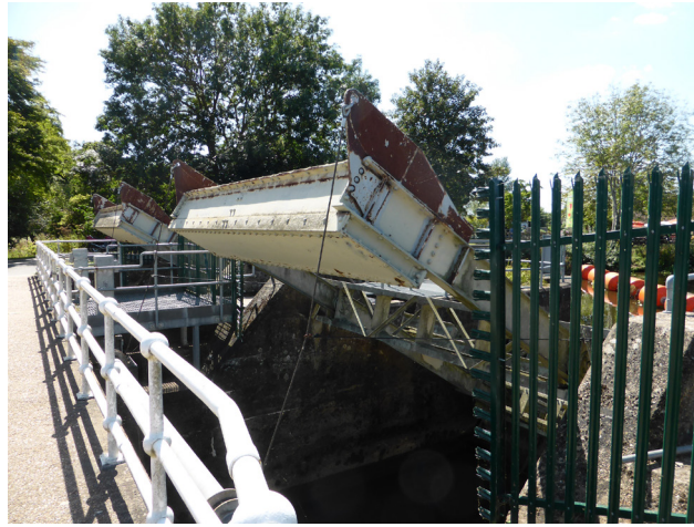
3. Radial sluice gates from road bridge
