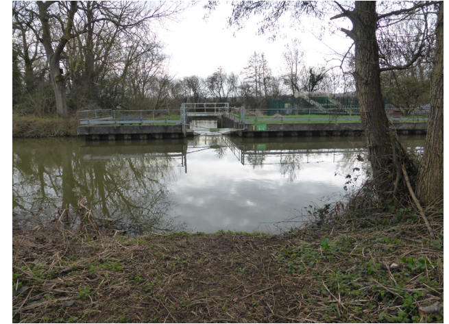
5. Weir with sluice & canoe and fish pass
