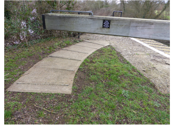
5. Grass lock-side with concrete heel grips
