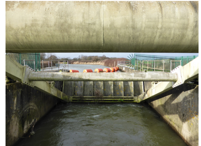
6. Sluice with radial gate
