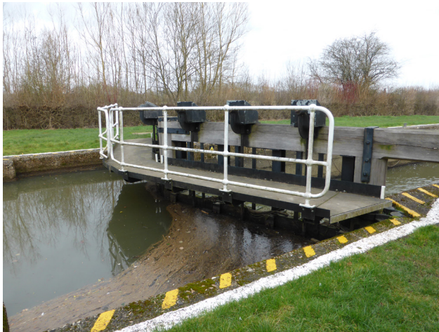
2. Head gates with x 6 gate paddles
