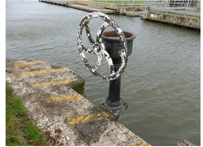
5. Disused ground paddle gear
