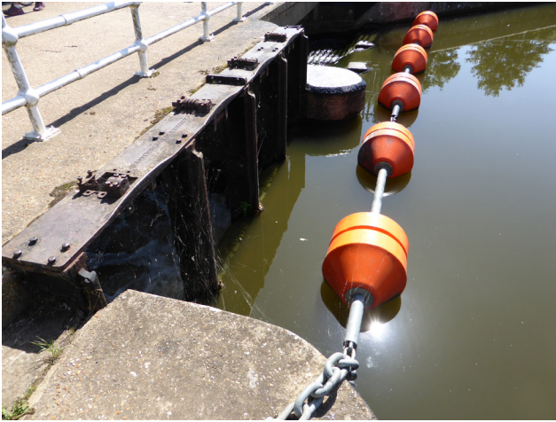
1. Disused vertical gates & fixed weir
