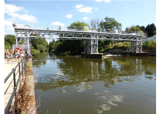
5. Two sluice gates
