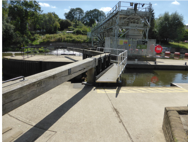
3. Tail gates with x 6 paddle gears & dated beam
