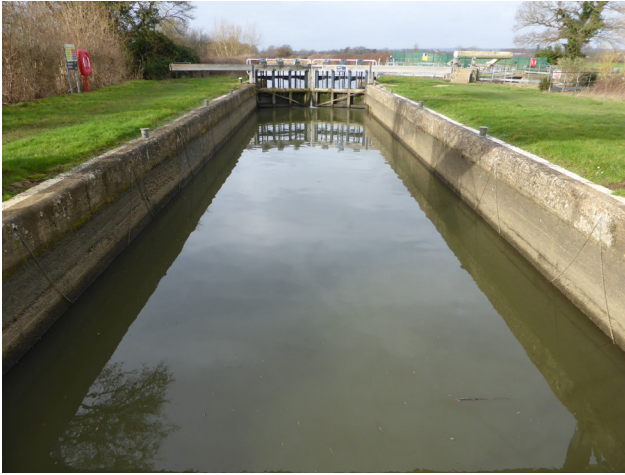
1. 1911–15 concrete lock chamber
