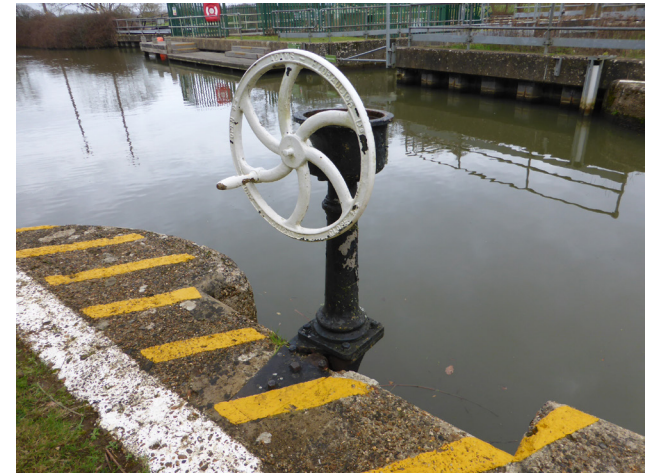
6. Disused ground paddle gear
