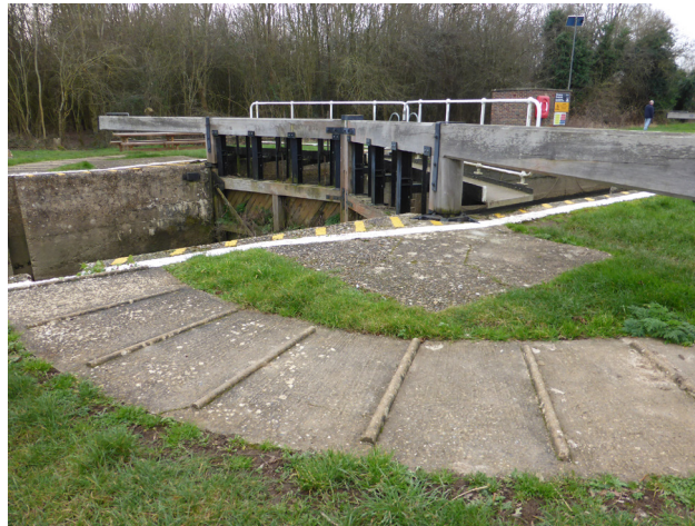
4. Grassed lock-sides with concrete heel grips
