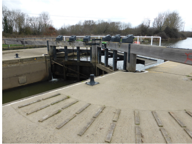
3. Head gates with gate paddle gears
