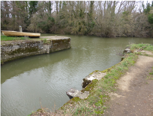
2. Remnant ground paddle gear and gate recesses
