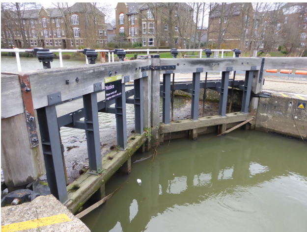
2. Head gates with paddles closed
