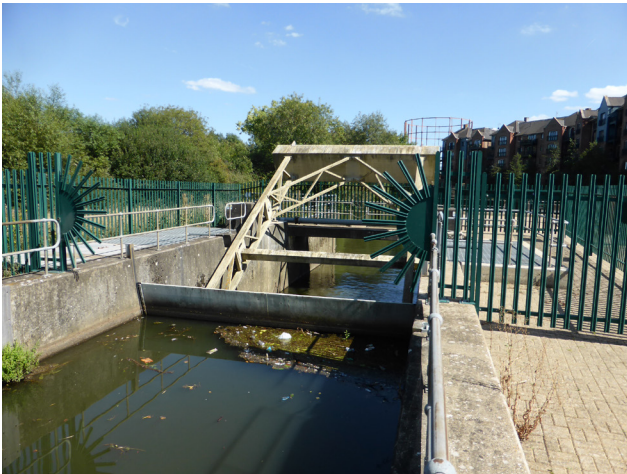
8. Radial sluice gate
