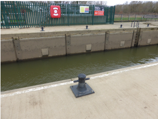
2. Concrete chamber & lock-sides
