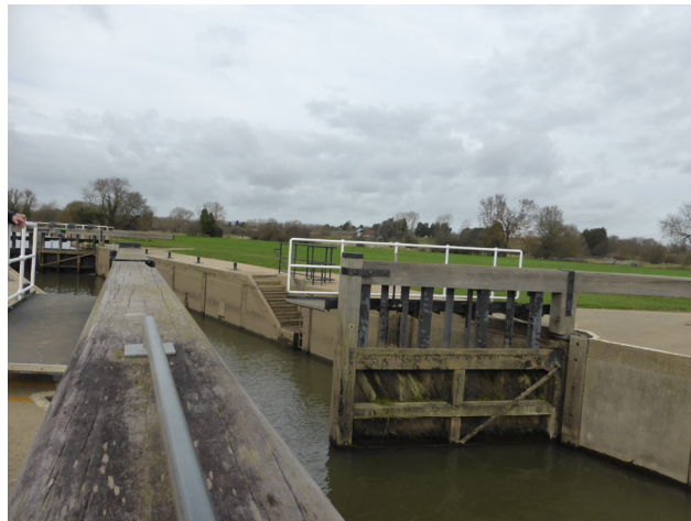
4. Tail gates with view towards chamber steps
