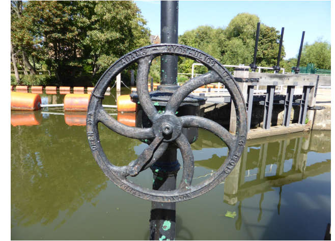
5. Disused ground paddle gear
