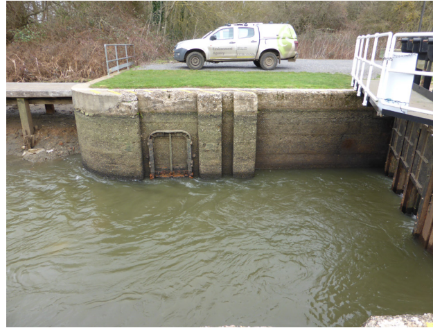
3. Disused ground paddle recess
