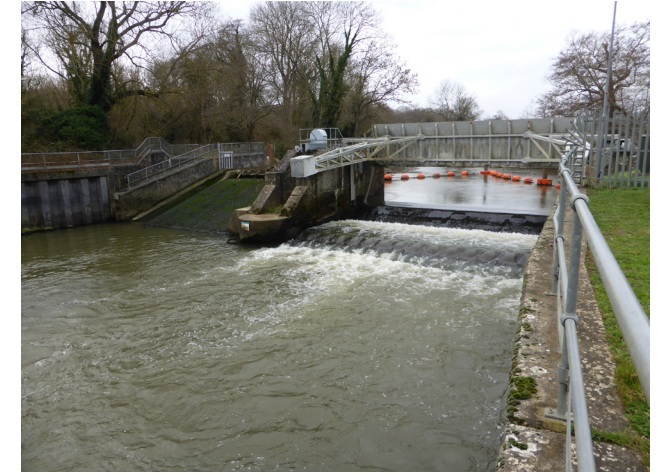
5. Weir with radial sluice gate
