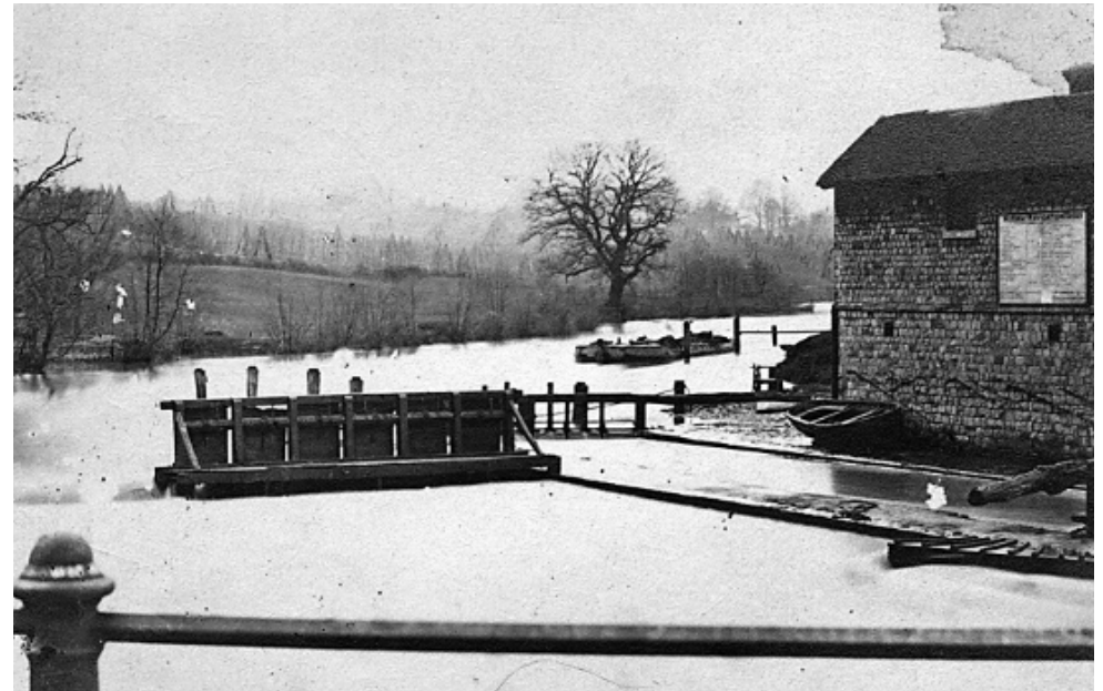
College Lock and Weir (of simple sluice gates). Note building on right with notice board displaying Upper Navigation Tolls (Maidstone Museum Archives, OMR5089).
