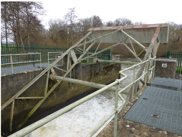
8. Sluice with radial gate
