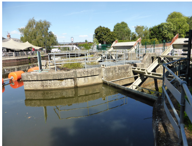
4. Radial gates & concrete buttresses
