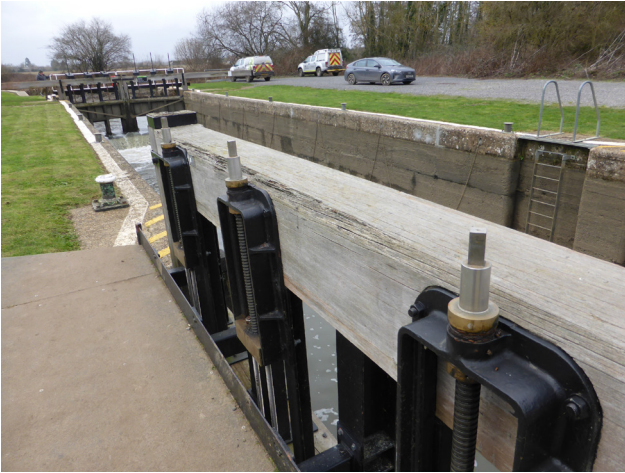
1. 1911–15 concrete lock chamber from tail gates
