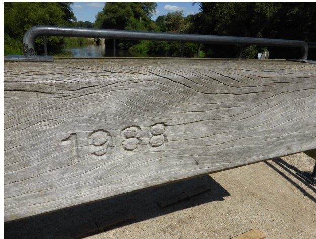
4. Dated balance beam on tail gate
