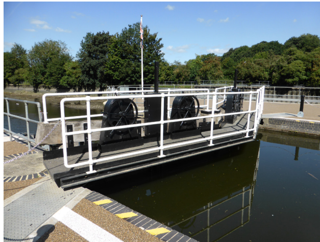
4. Preserved paddle gear on tail gates
