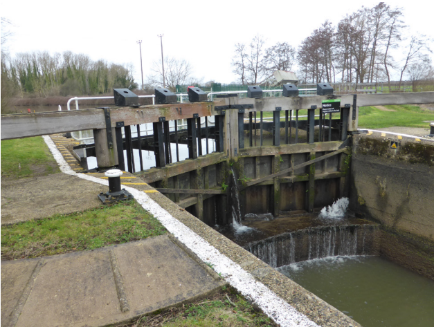
2. Head gates with gate paddles
