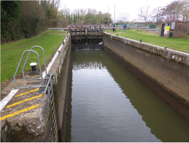
1. 1911–15 concrete lock chamber
