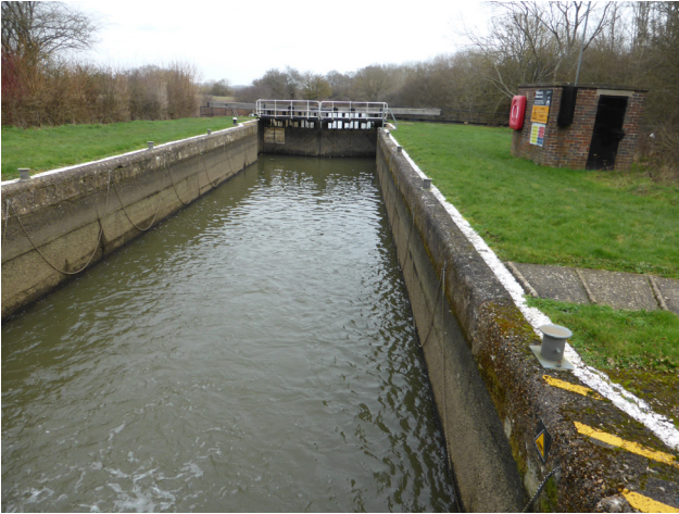
1. 1911–15 concrete lock chamber
