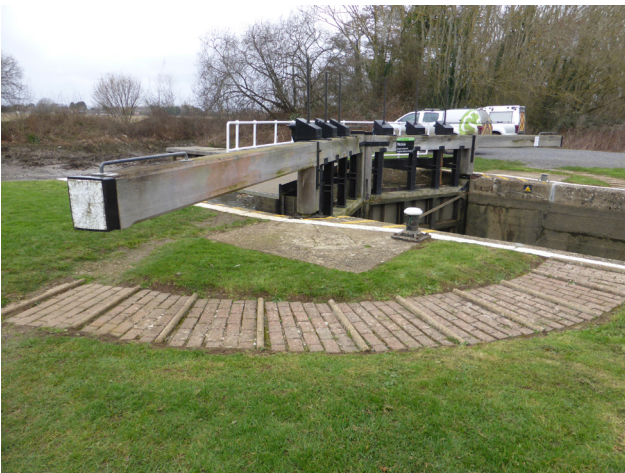
2. Head gates with concrete heel grips
