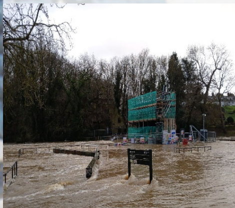
Teston during heavy rain fall in January 2025
